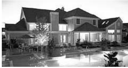
The Village Green at Cantera development is an upscale residential community with resort-class amenities located in Warrenville.
