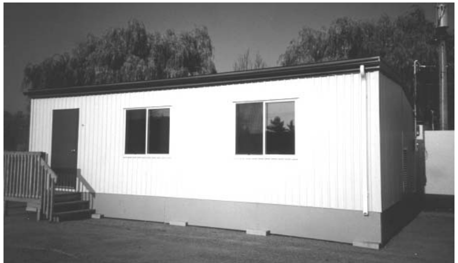
Portable classrooms like this one may raise air quality concerns without proper ventilation and maintenance.
