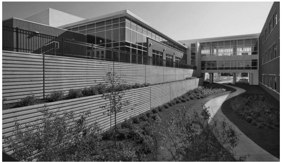
Award-winning Hubble Middle School in Wheaton Warrenville CUSD 200, designed by Legat Architects, was a key stop for a touring green building conference recently.
